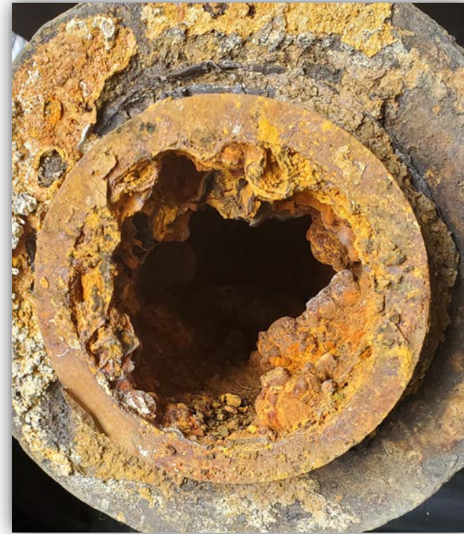
Sediment Buildup & Corrosion of Aging Waterlines (5 Year CIP includes replacing similar condition waterline on Quincy Boulevard and 4 th Street Terrace)
